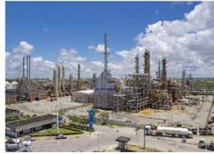
Braskem VCM plant (Photo courtesy of Braskem)
