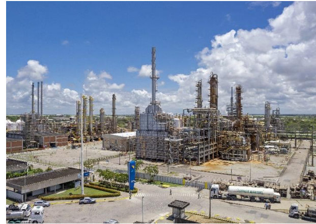
Braskem VCM plant (Photo courtesy of Braskem)
