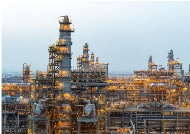
Saudi Aramco's Fadhili Gas Plant (Photo courtesy of Saudi Aramco)
