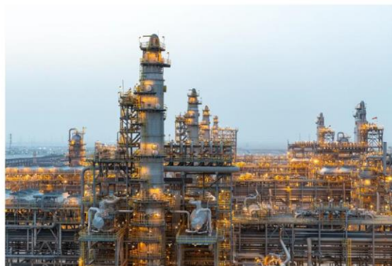
Fadhili Gas Plant (Courtesy of Aramco)
