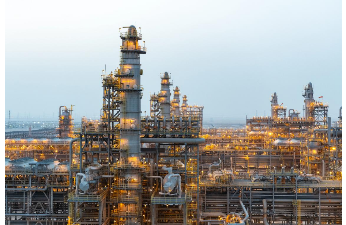
Fadhili Gas Plant (Courtesy of Aramco)
