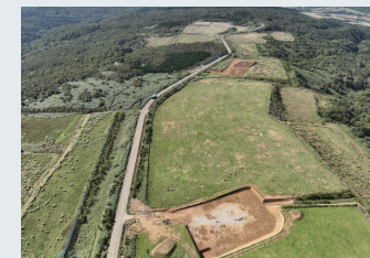
Planned construction site of the Shimamaki-Kuromatsunai Wind Farm (Photo courtesy of Cosmo Eco Power Co., Ltd.)
