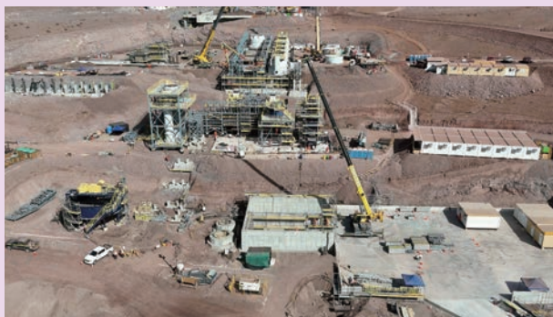
Minera Arqueros plant under construction The commercial operation is scheduled to start during FY2026 (Taken in May 2025; photo by Compañía Minera Arqueros S.A.)
