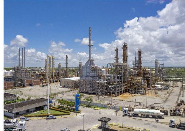
Braskem VCM plant (Photo courtesy of Braskem)
